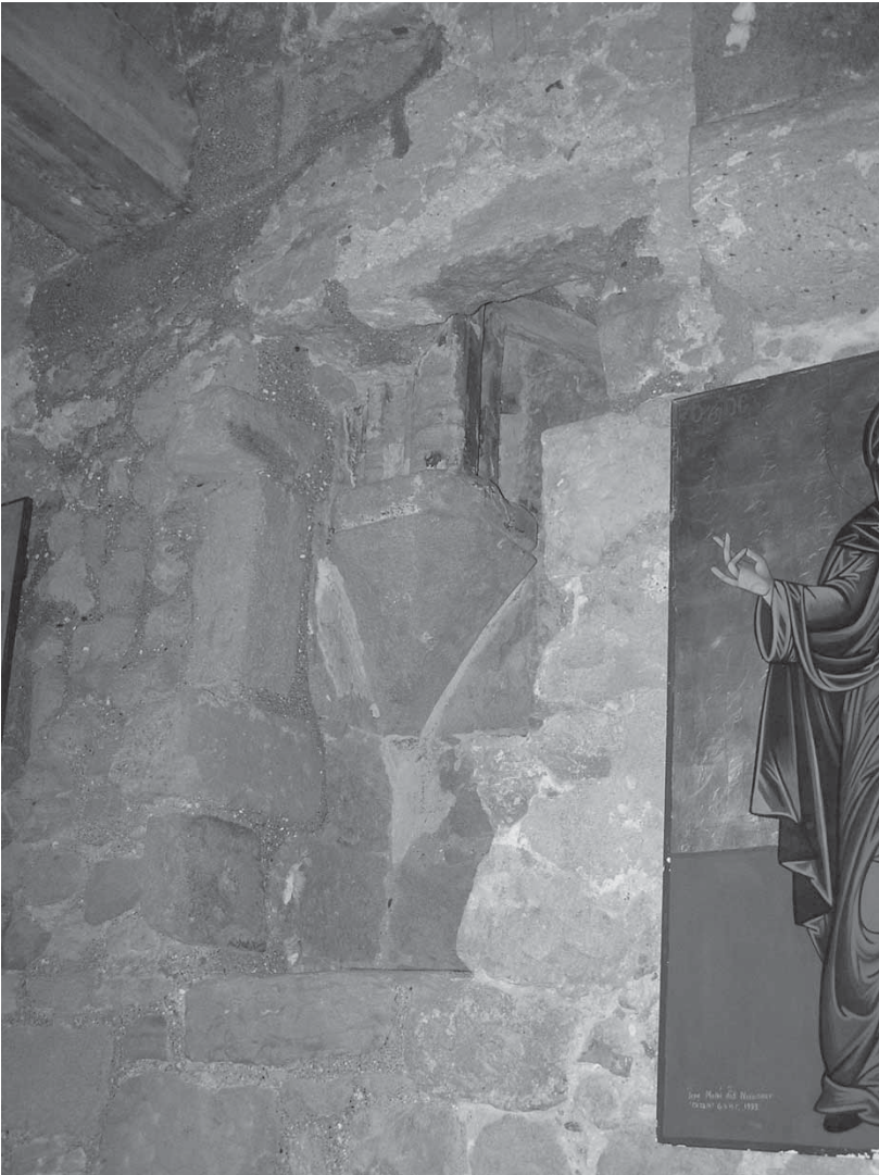
Fig. 68: St Nicholas of the Cats, church, corbel and rib spring brought to light within the present thickness of the south wall [M. Olympios].
